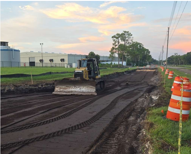
Webster Turn construction
